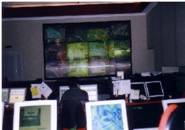
Plate 1.8: The Traffic Control Centre Rome.
