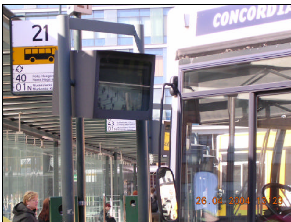
Plate 2.10: Rear view screens to enable safe negotiation of the bus loading areas
