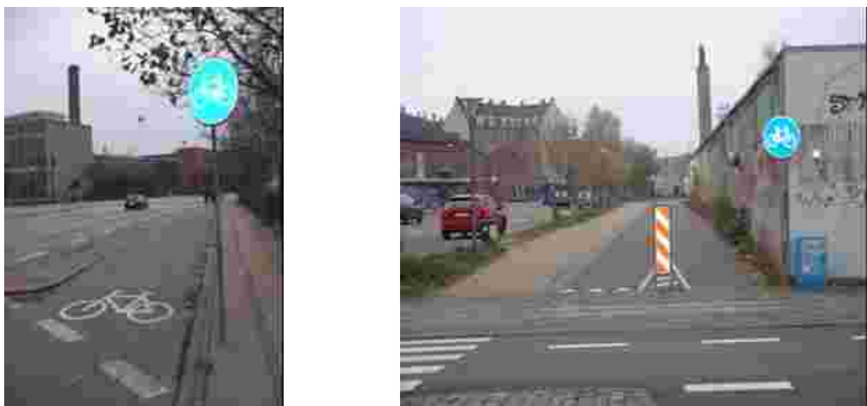
Figure 3.12 and 3.13: Greenways are segregated form the roadspace through street furniture and signage
